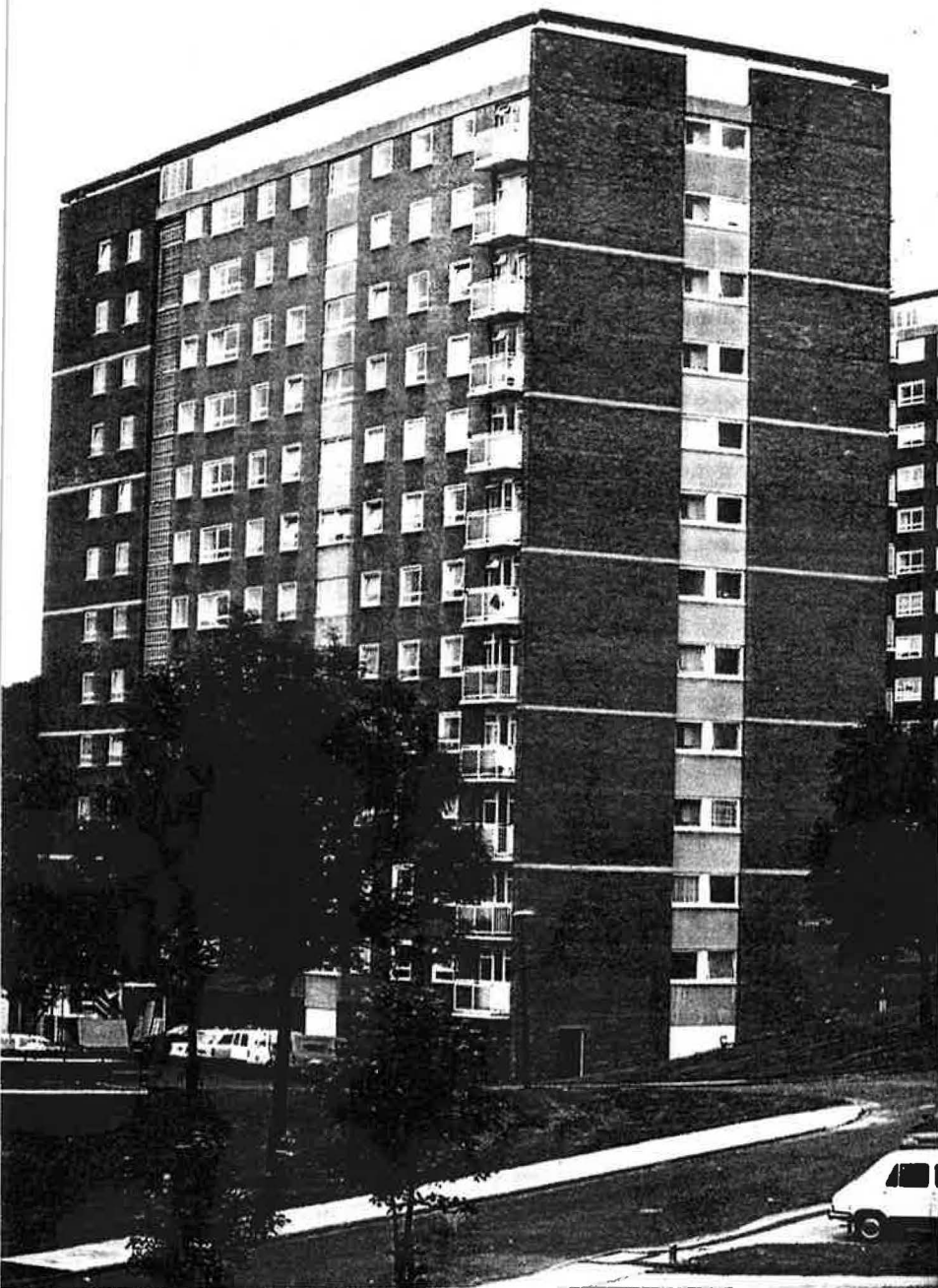
The Sandwell high rise flats
