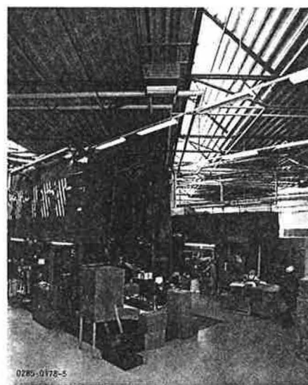
5 Plastics production in an Austrian works fitted with ceiling mounted recirculated air heat exchangers.
