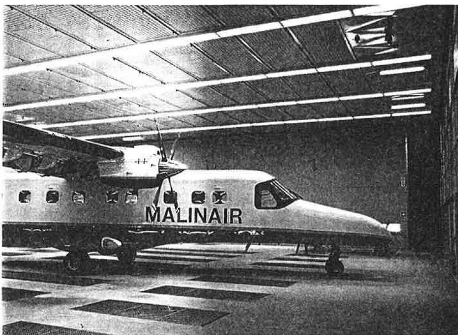
19 Lacquering hall of an aircraft manufacturer in the Federal Republic of Germany. The air handling is program-controlled (filter ceiling, below — air extract via floor grid complete with paint mist separator).
