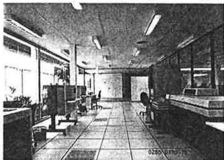
9 Microfilm production room with floor air outlets (source ventilation). The cooling air is supplied to the machines directly via perforated floor tiles and rises to the ceiling.
