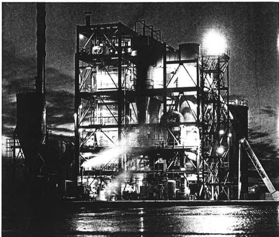
View of 50t/h Multi Solid Fluidised Bed boiler plant at Listowel, Republic of Ireland.
