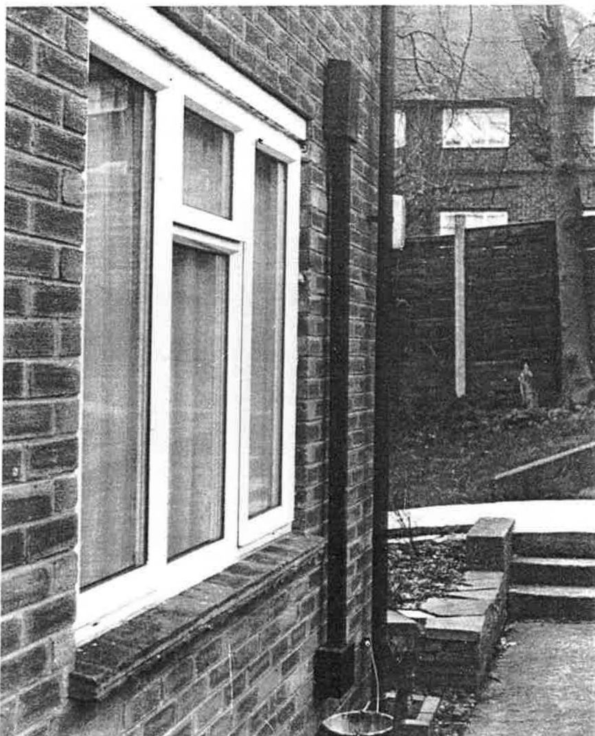
Figure 3: A typical 'Good Health' system on a house.
