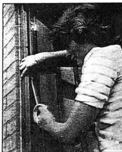
A member of the DPAA applying draught proofing material.
