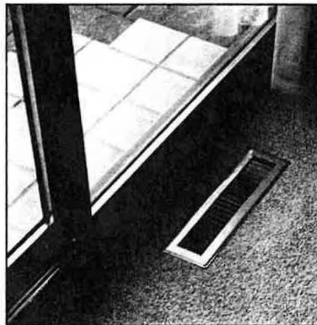
Discreet floor grilles can be used to distribute warm air.
