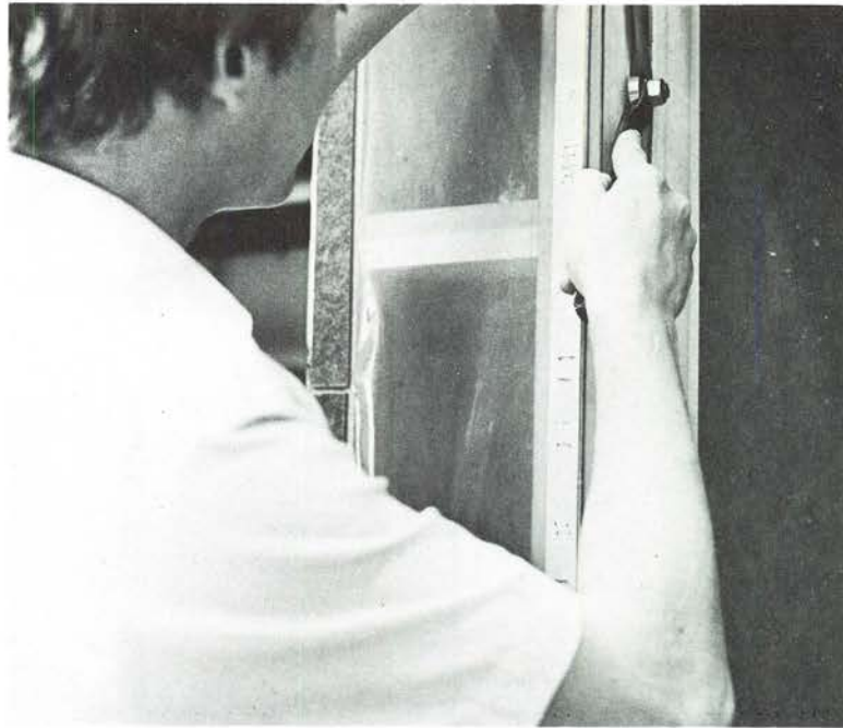
FIG. 22. Mounting of weather-strip with toe in the groove. The tool is a ball bearing with a handle.
