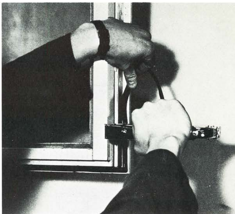
FIG. 14. Mounting of weather-strip with staples onto window casement without a groove. According to HusAMA (Material and Workmanship Specifications for Building Construction), the spacing of the staples is to be 80 mm. In some cases work is made easier if the casement is taken off.
