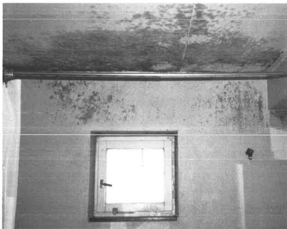
Damage caused by damp beneath a roofing structure. This damage has been caused by a high humidity level in combination with poor insulation in the attic. Photo: Rune Pehrsson, Familjebostäder, Stockholm.
