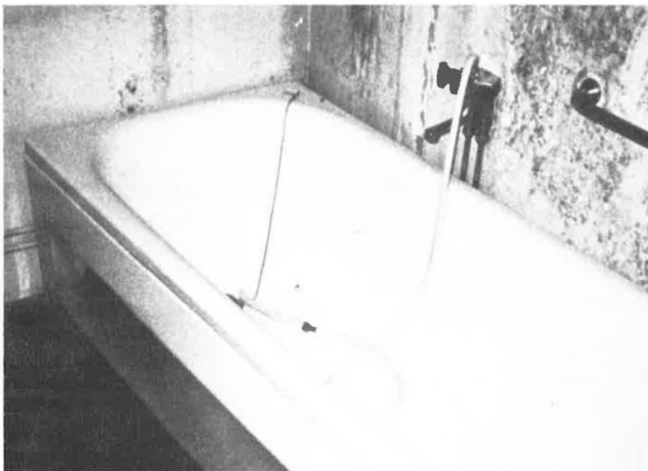
Severe mildew damage to bathroom walls. The walls have been painted with water-based latex paints on glass-fibre fabric. Photo: Rune Pehrsson, Familjebostäder, Stockholm.
