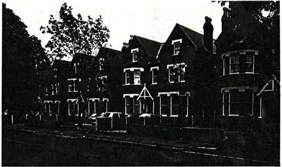
Energy Efficient Housing Refurbishment. Many older houses can have their energy performance upgraded when they are re-furbished.
