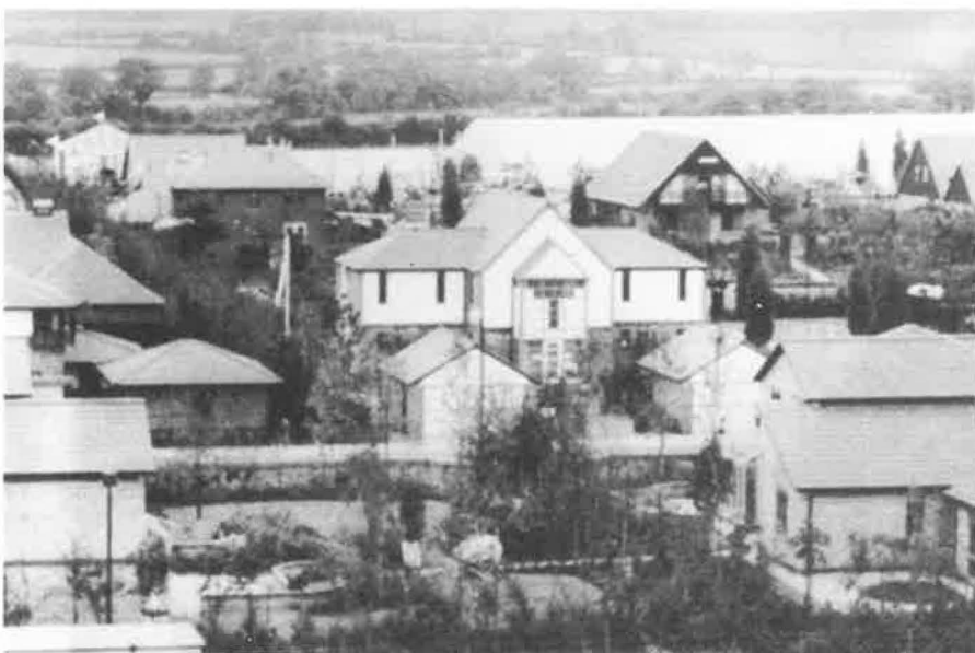
Milton Keynes Energy Park
