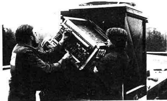
Fig. 5: The cooling coil is placed in the exhaust air unit.
