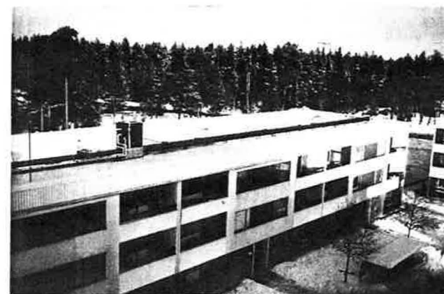
Fig. 3: Test house in Gävle. Exhaust air unit and duct system visible on the roof.
