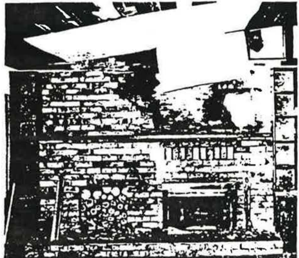
← Photo 2 This case occurred in Prince George on December 18, 1983. A heat exchanger unit with glass doors (manufacturer calls it a converter furnace) was installed a year ago into a masonry fireplace that was built 15 years ago. The unit was listed by Warnock Hersey Professional Services Ltd. Clearance between the sheathing and the chimney appeared to be almost nil and insulation between the sheathing and panelling might have compounded the problem by restricting the dissipation of heat.
