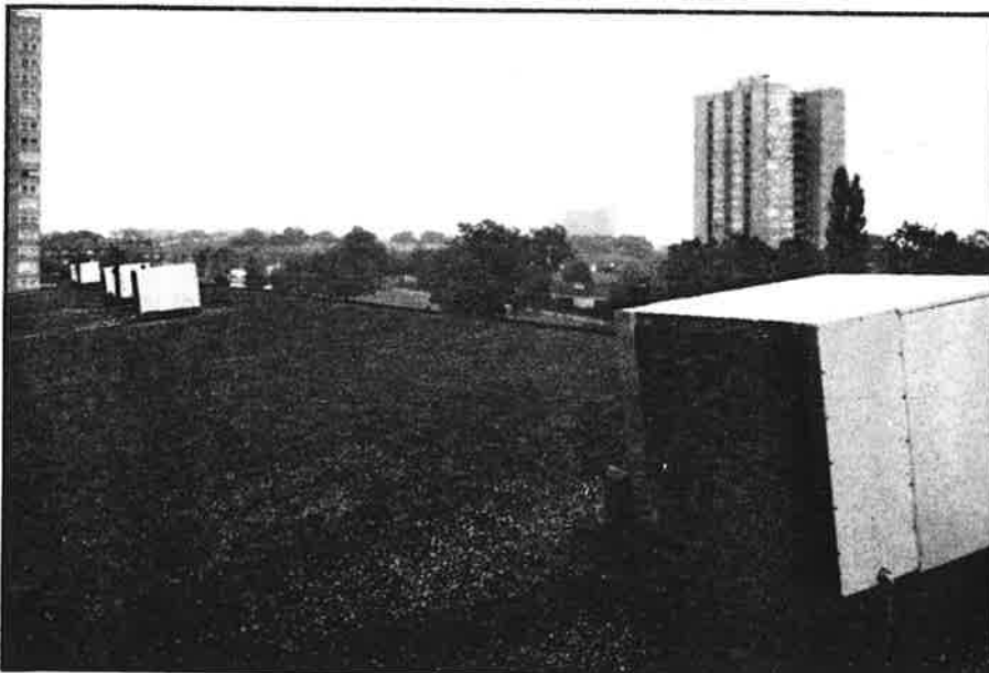
3-in-1 Ventilation Savers.....compact roof mounted units at Stevenage: each unit simply installed, saves space, cuts energy cost through air handling, VAV and heat recovery (ESG Controls, Cambridge)
