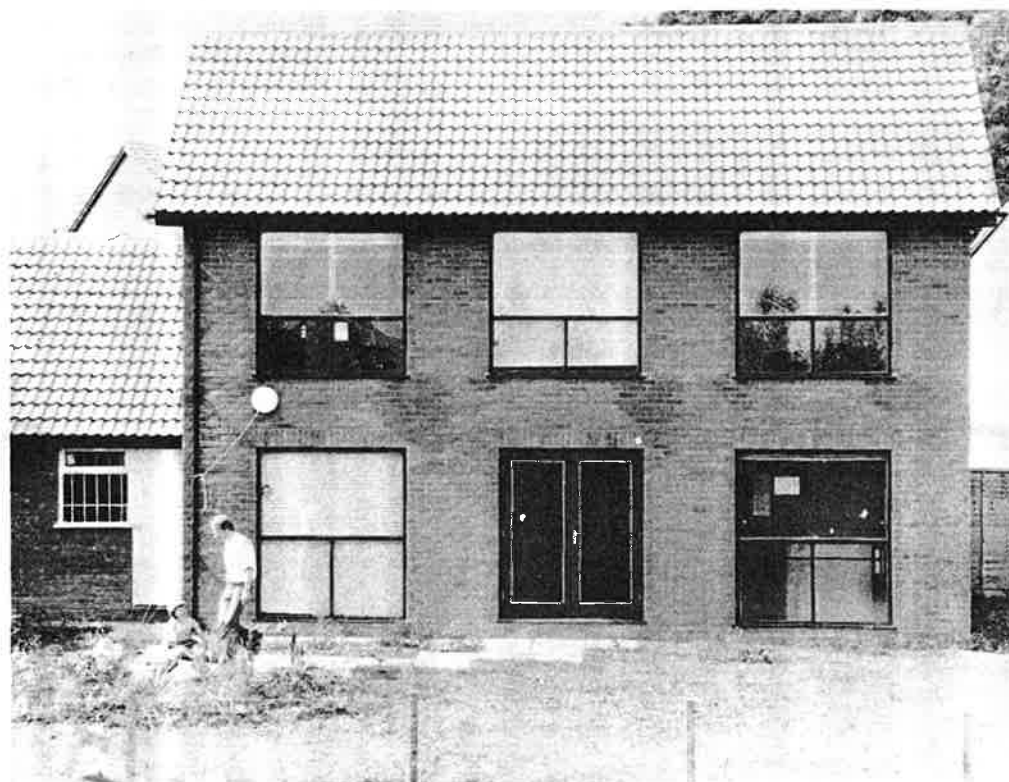
Figure 3 Large south-facing glazing on Linford houses.
