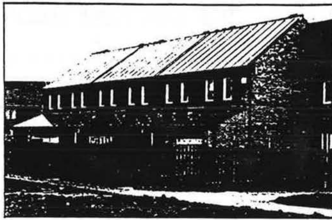
2.2.1 Monitored low energy house at Peterborough
