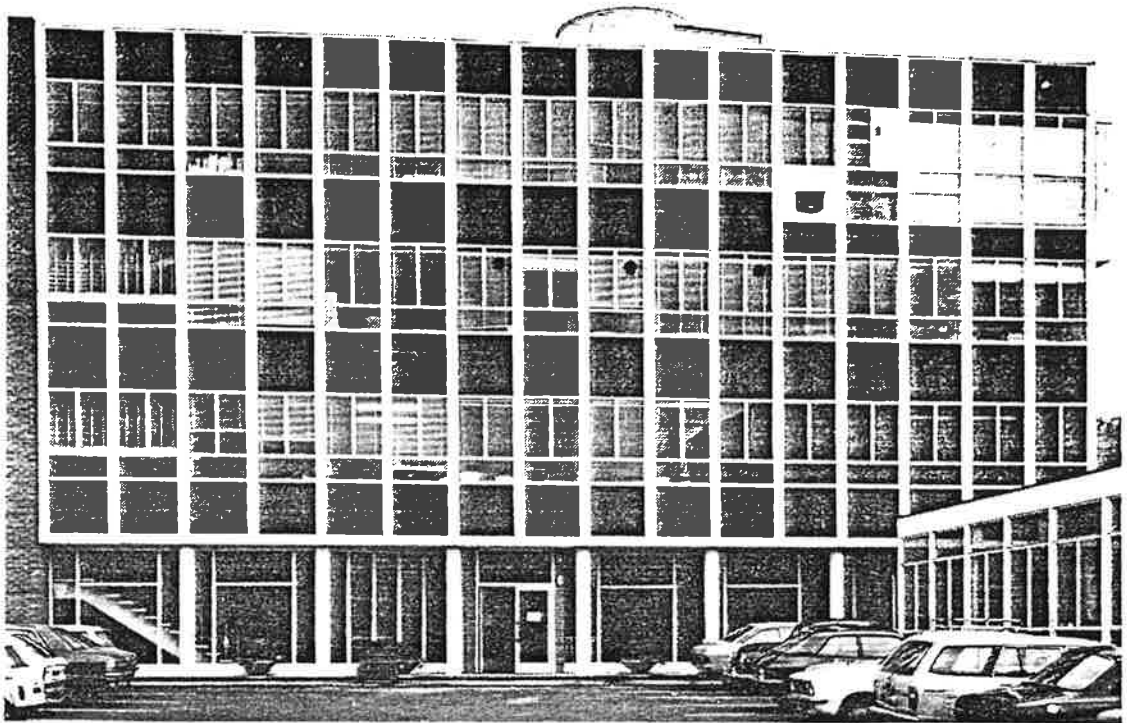
Figure 7 South face of building B
