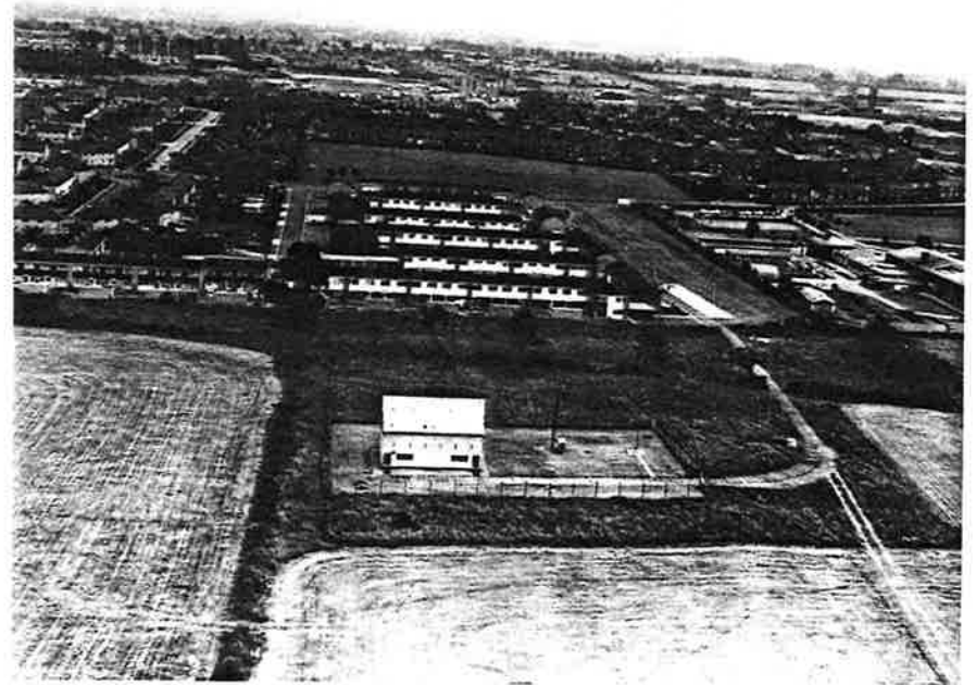
Fig. 1. Aylesbury site looking East.
