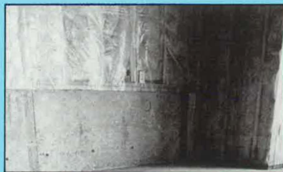
Carefully poured and sealed concrete slabs help block the entry of radon into the home.
