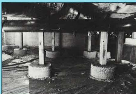
Preventive measures, such as placing ground covers over exposed soil in crawl spaces, help block the movement of moisture into the home.
