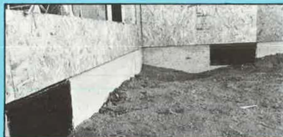
A well-ventilated crawl space allows radon to escape outdoors, rather than enter a home.
