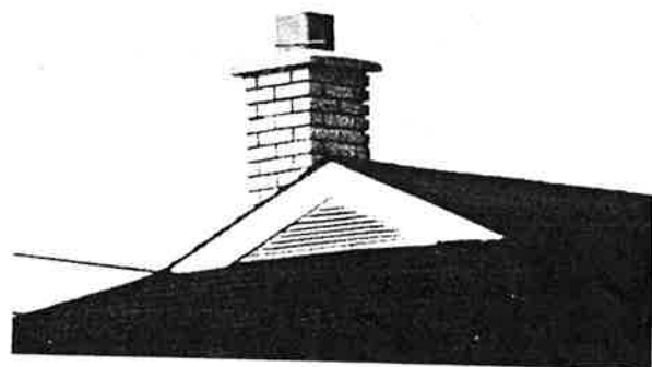
Figure 11. Triangular vent near the ridge of a hip roof
