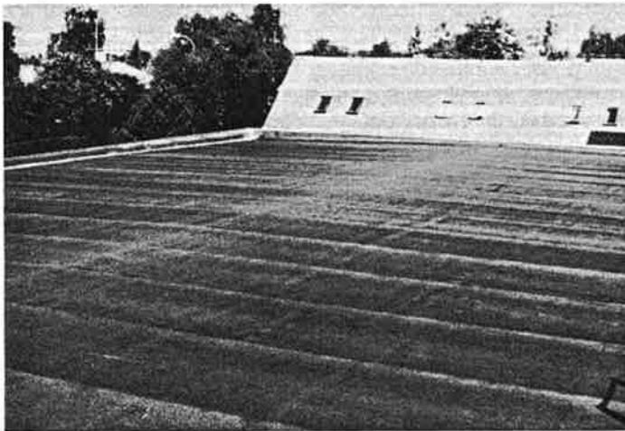
Fig. 9. View of the new 'warm' roof: all roof vents have now been removed
