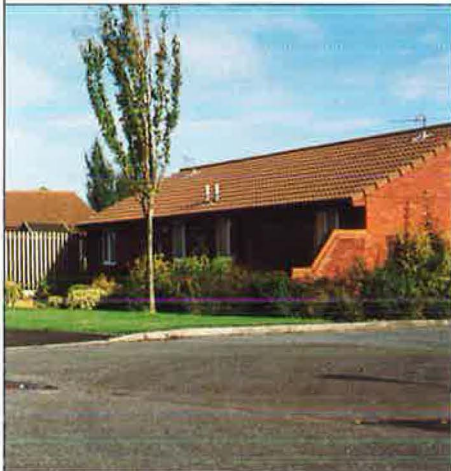
Passivent PSV-M systems have also been installed by Warrington Borough Council in their refurbishment programme.
