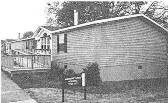
Figure 2 — Palm Harbor's new prototype (left) sits next to an ordinary model on the campus of North Carolina Agricultural and Technical State University. The two manufactured houses will be monitored for a full year.
