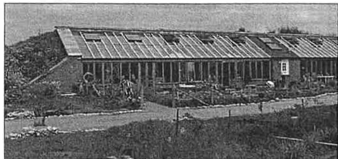
Figure 14 — The Hockerton Housing Development is a zero-energy, earth-sheltered housing scheme pointing the way for future developments. Several similar schemes are now under way.
