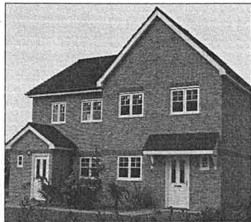
Figure 13 — A semi-detached pair of houses assembled from volumetric units (four per house) and built in a week. The developer wanted a traditional look so they were clad in brick tiles to look like traditional brickwork.
