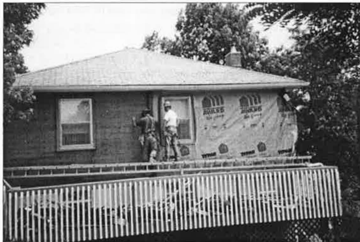
Exterior air barrier being installed
