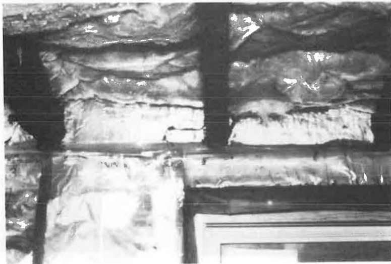
Figure A-5. Air/vapor barrier between floor joists. Polyurethane boards were put between joists and caulked to them and to the flooring above. The wall air/vapor barrier ends on the bottom of the floor joists.
