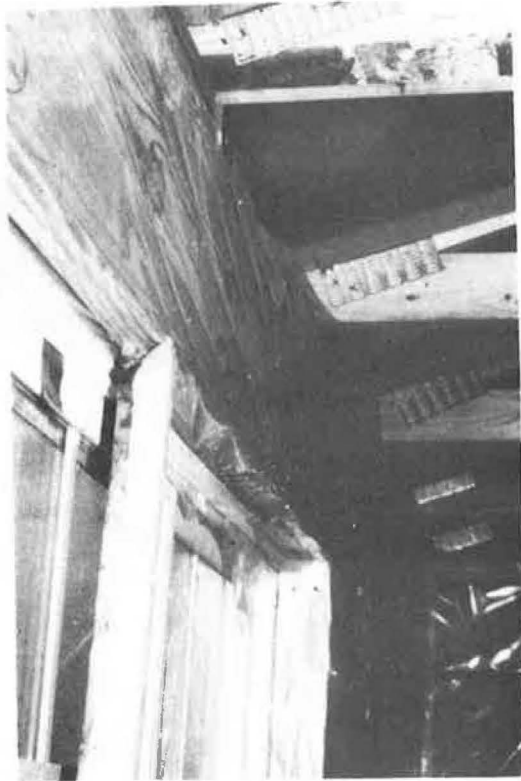
Figure A-26. Technique for sealing air/vapor barrier to window by clamping with a molding piece.
