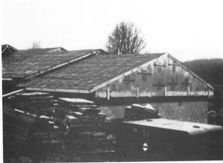
Figure A-33. Townhouse floors and roofs are built right on the foundation, lifted off at the time walls are erected, and then put back in place.
