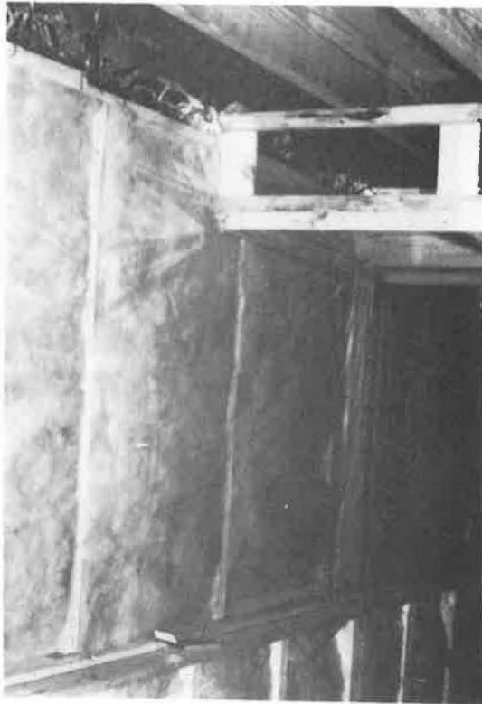
Figure A-29. Insulation and air/vapor barrier inside basement wall, for living space.
