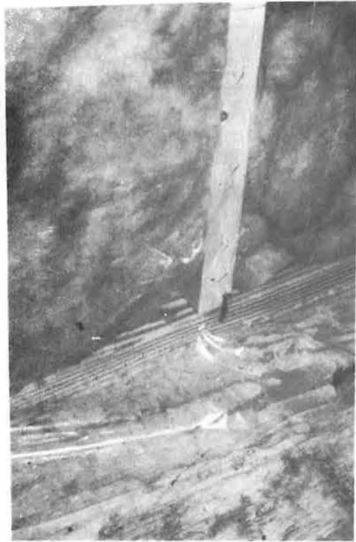
Figure A-25. Sealing of sill with an open-cell foam strip, also used between construction elements. Note the air/vapor barrier's overlap into the floor.
