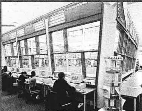
RIGHT: The student workstations overlook the central lightwell, the high-level dampers are visible at the top. FAR RIGHT: A section showing the central lightwell and perimeter exhaust stacks.
