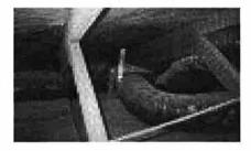
You should be aware that you only need to insulate ducts that are in unconditioned or partially conditioned spaces. These areas include: attics, garages, basements, and crawlspaces.
