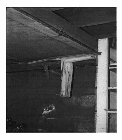
The picture above is an example of loose duct tape on a return duct in a basement leaving a sizeable hole for unconditioned air and dust to enter the forced air system
