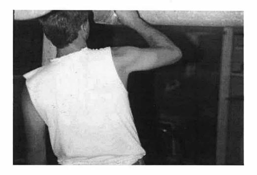
Openings frequently occur at the joints of duct segments. By applying generous amounts of mastic around all of the joints, you can stop the flows of air out from the supply ducts and into the returns. In the photograph above, a weatherization specialist is applying mastic with a brush to the joints of a supply duct.
