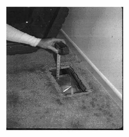
It is often rather easy to remedy this problem; pull the boot up to the floor and attach it securely or extend the sheetmetal to meet the floor. In either case, one must then seal the boot so that the air that the fan blows is actually delivered to the room. The picture below show a boot being sealed to the floor.
