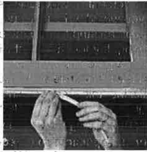
Rubber bulbs and seals are effective for sash window bottoms, but may require power tools to cut the kerf that holds the barbed flange.
