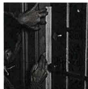
You can make a stop and seal combination by kerfing stop moulding, then adding a barbed seal. Install so the seal is compressed 20% to 30%.
