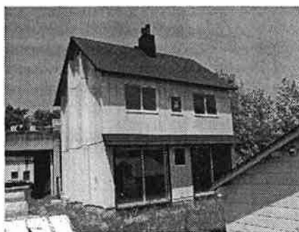
Photo 1: The Full-scale Test
