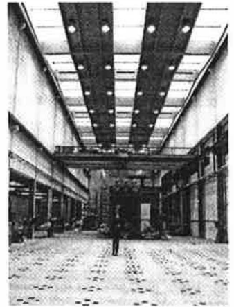
Figure 1: Picture of the laboratory hall with the glazed roof during retrofit work
