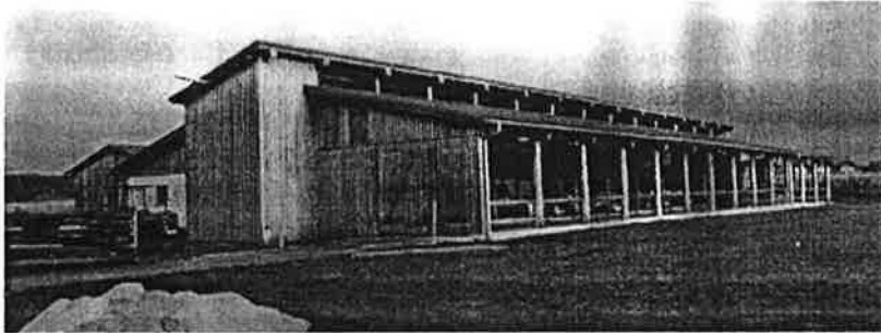
Fig. 3: Front opened livestock building with spaceboard (enclosed space: 3411 m 3 ; number of animals: 74)
