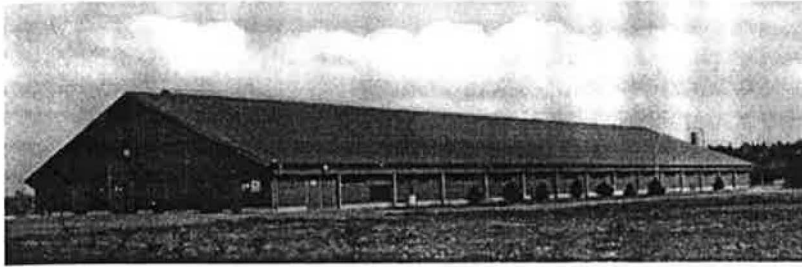
Fig. 2: Livestock building with eaves/ridge ventilation (enclosed space: 10694 m 3 ; number of animals: 225)
