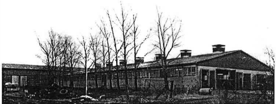
Fig. 1: Livestock building with shaft ventilation (enclosed space: 5445 m 3 ; number of animals: 202)
