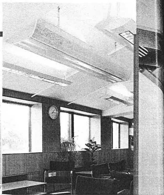
LEFT: One of the cellular offices, and RIGHT, an open plan area. Passive infrared presence detectors fitted to the inner lights can be set up to control the lamps, but this has not proved popular.
