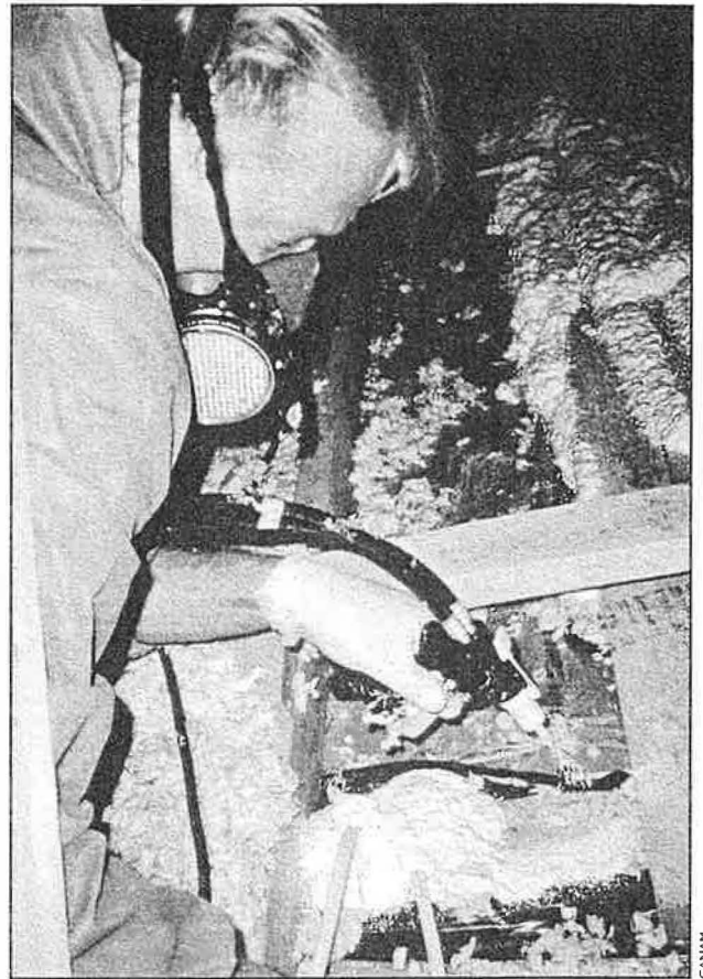
The crew lays continuous beads of foam to seal all leaks.
