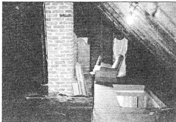
The attic room before remodeling changes were made.
