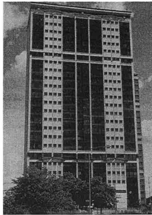
Figure 2 Multistorey block after refurbishment
