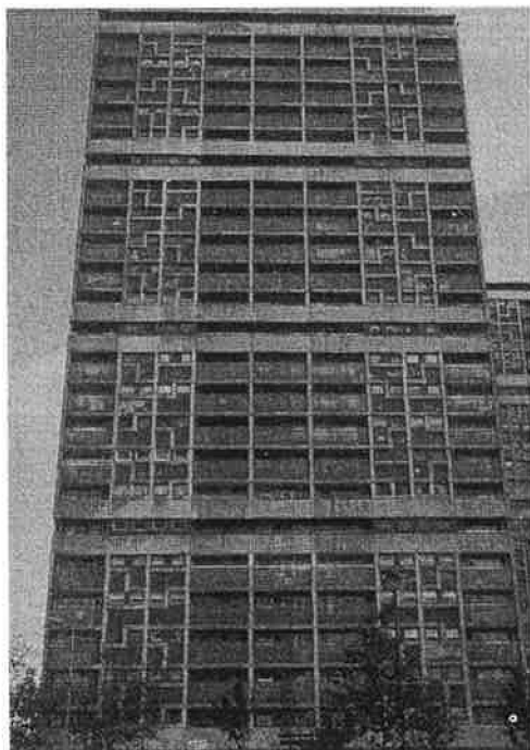
Figure 1 Multistorey block before refurbishment
