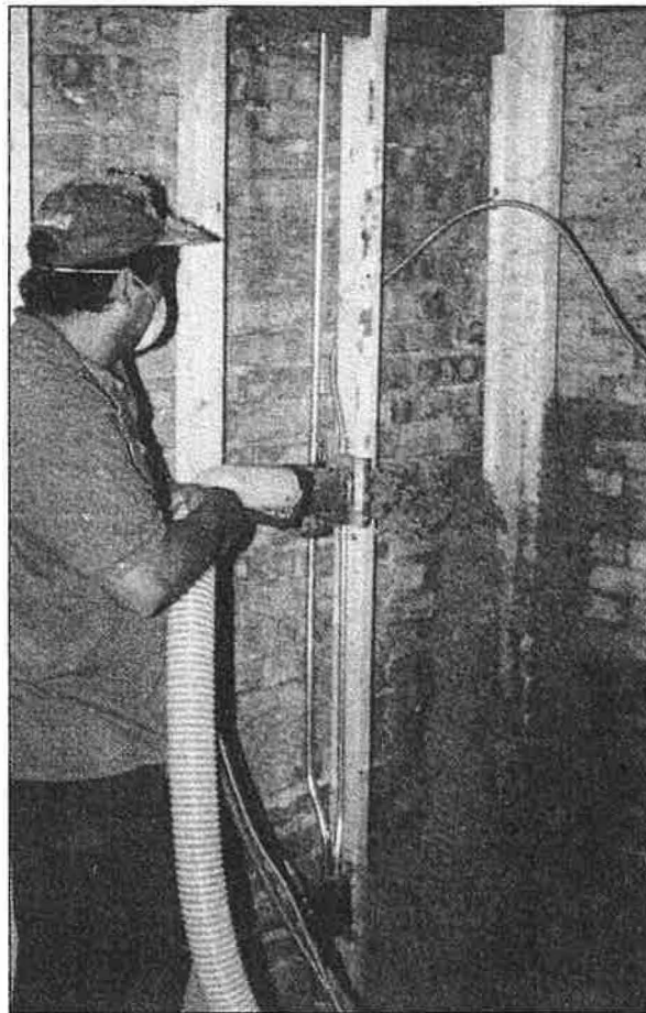
Spray rock wool was used to insulate the exterior walls.
