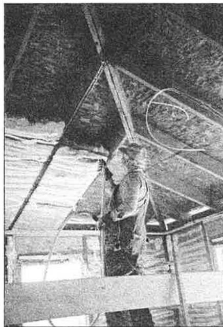
A contractor is insulating this ceiling with Airkrete.
