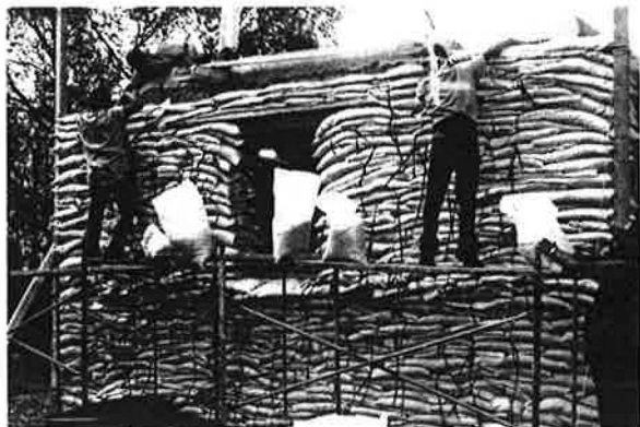
Figure 1 Pumice wall in construction.
