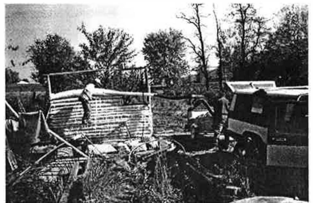
Figure 7 Sawdust wall under construction.
