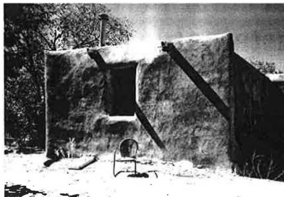
Figure 2 Pumice wall after three years.
