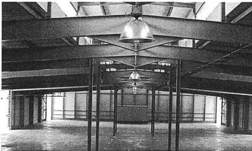
ABOVE: The 87 m x 38 m production area of the factory unit. Note the lack of support columns and the light available despite the lamps being uninstalled. LEFT: Roof level windows are used to increase daylight levels and as part of the ventilation strategy.
