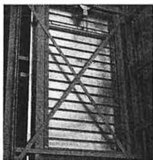
ABOVE: The factory's natural ventilation strategy at the design stage. Note the full glazing of the 'pop-ups', this was later reduced on cost grounds. - RIGHT: A ventilation louvre viewed from inside the production area.
