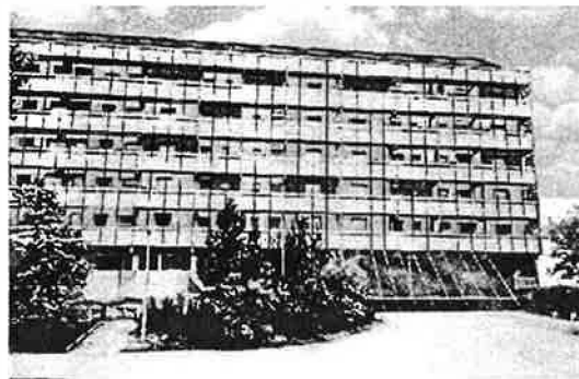
Fig.2 Building in Goteborg. Illustration: Christer Nordström
