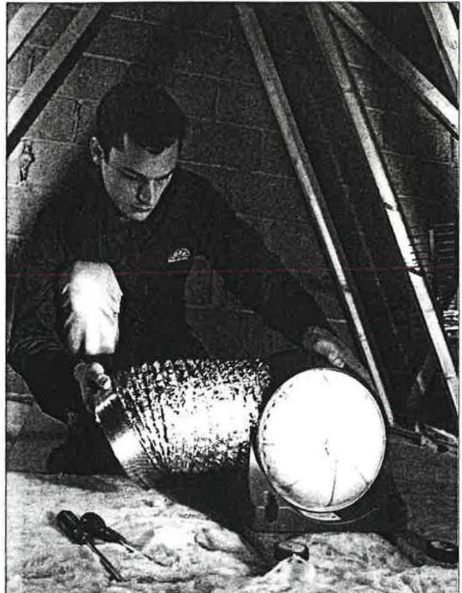
**FIGURE 1: A typical installation of a positive ventilation unit, in this case a Home Ventilation Drimaster 5 unit being installed in a roof space.**
