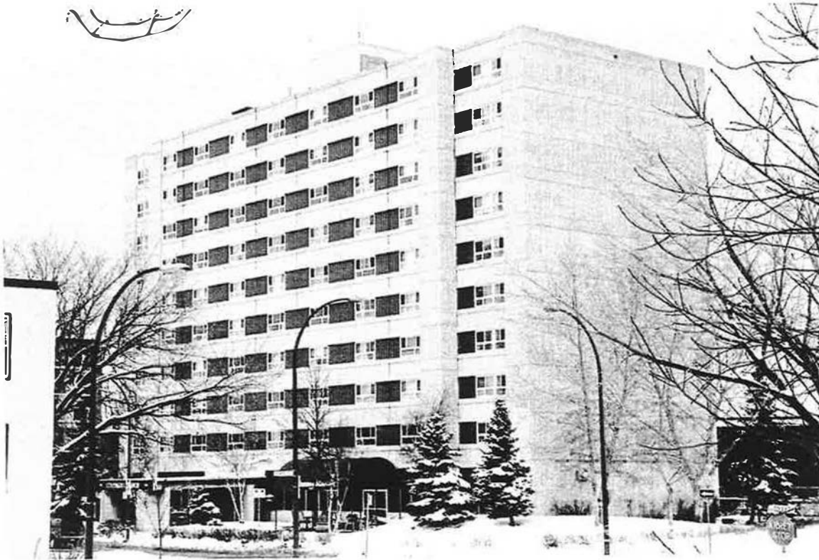
South and East Elevations
