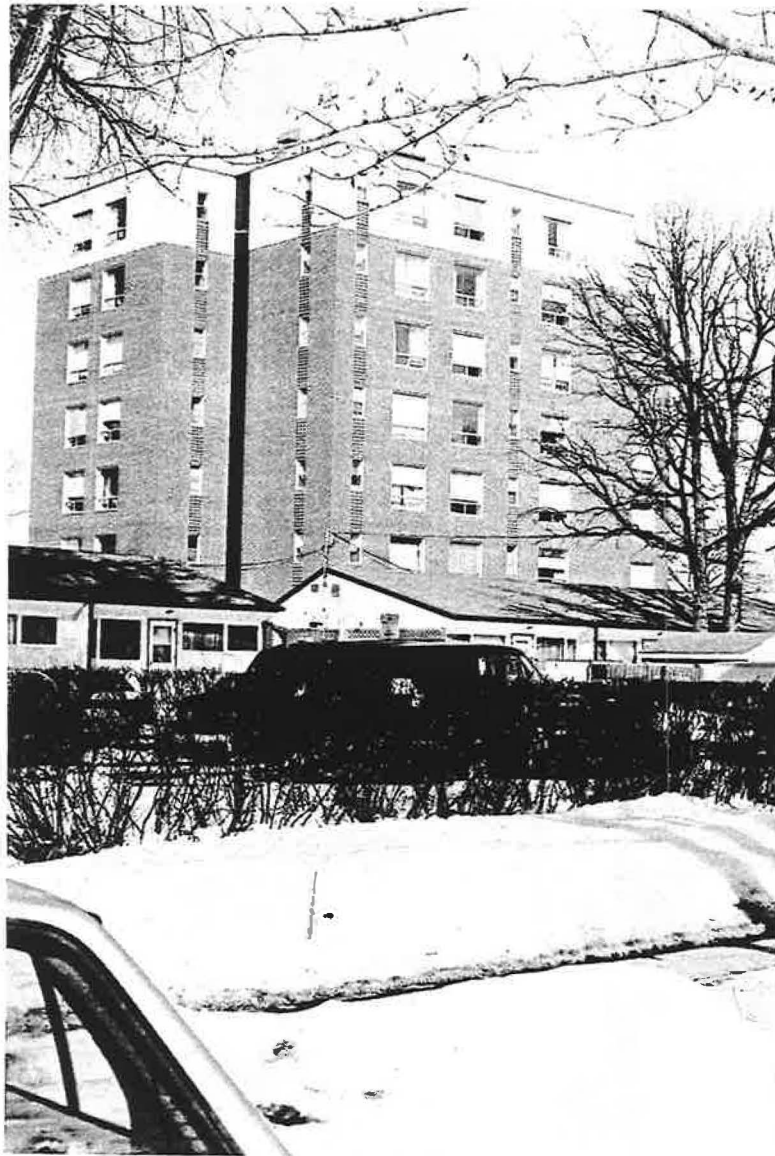
West and South Elevations
