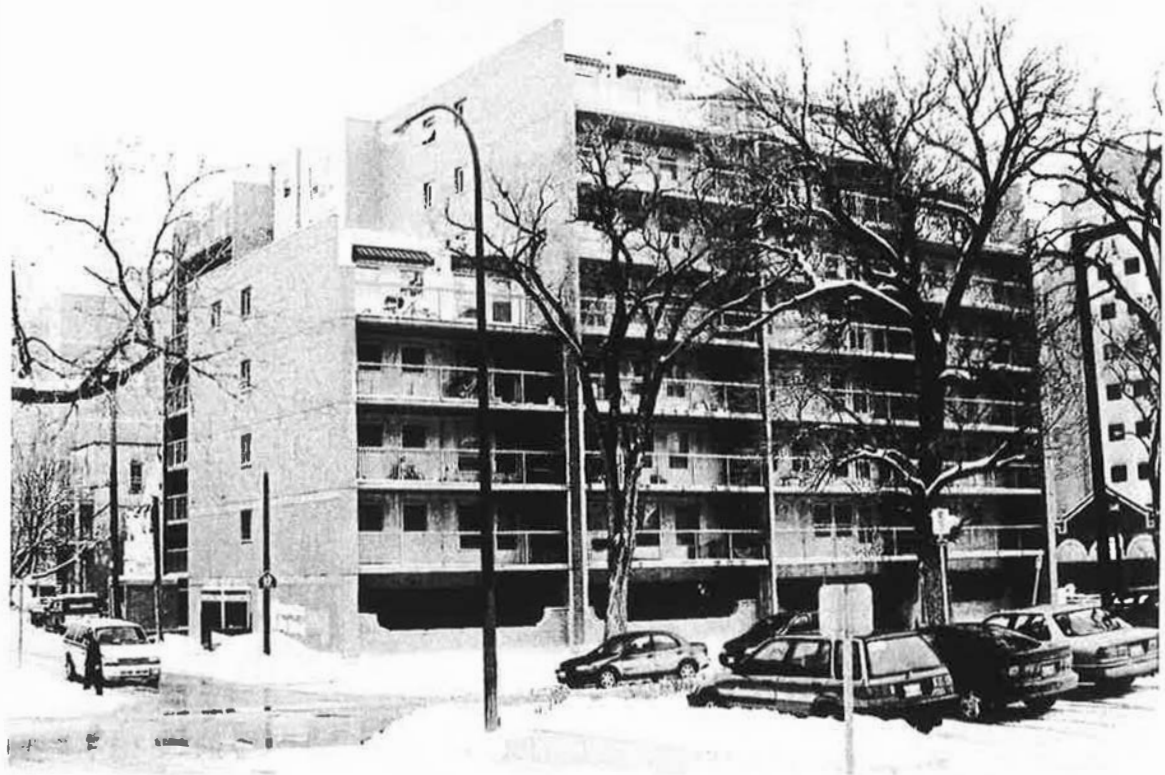
West and South Elevations
