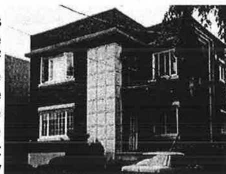
Figure 1: Case Study Building
