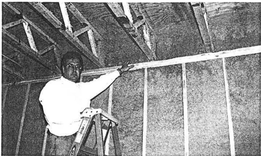
Jay Epstein's company, Gabriel Enterprises, uses advanced air sealing and high-density cellulose insulation to minimize a house's indoor/outdoor air exchange. Tests have shown that cellulose insulation reduces air exchange by 38%.
