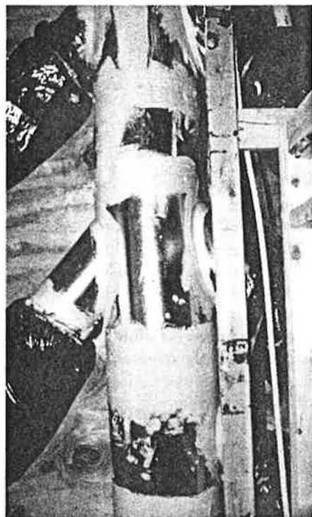
By installing a round main duct and angling peripheral ducts at 45°, Gabriel Enterprises improves the efficiency of its air handler.
