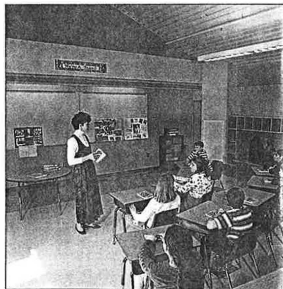
FIGURE 3. A typical classroom at Boscawen Elementary School showing a vaulted ceiling that facilitates displacement air flow.
