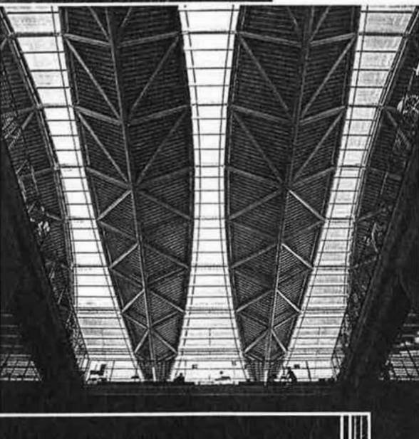
8. Butterfly wing roof trusses over the centre of ST1.
