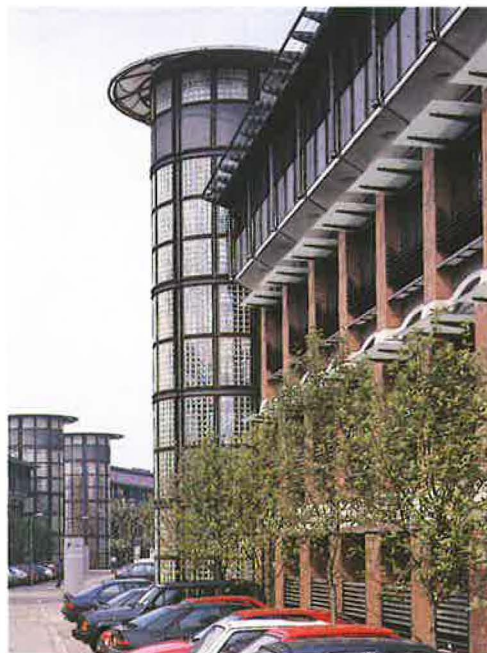
Figure 6 Inland Revenue Building
