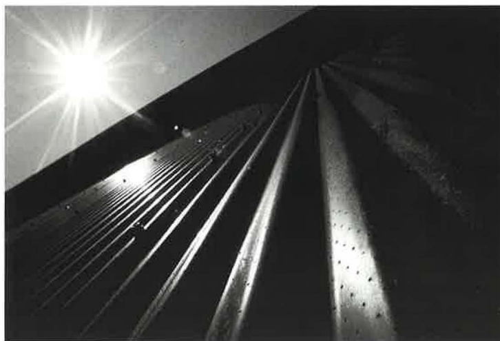
Solarwall showing perforated hole construction and canopy.
