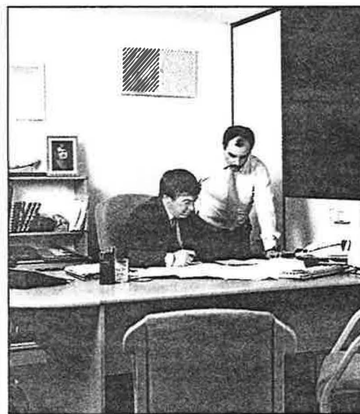
Modern through-the-wall ventilation units provide a balanced 2-way flow of air with energy exchange between the two airstreams. This is Vent-Axia's HR500.
