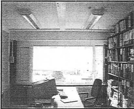
Figure 6a: Office at the west façade – large ventilation grilles and external screens
